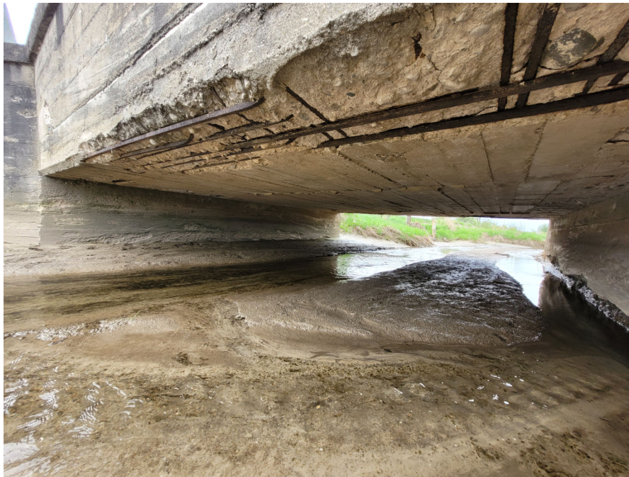
View of abutment wall and soffit, typical.
