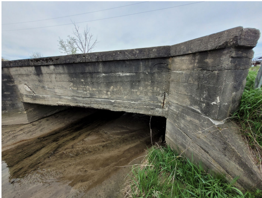
View of exterior of parapet wall, typical.
