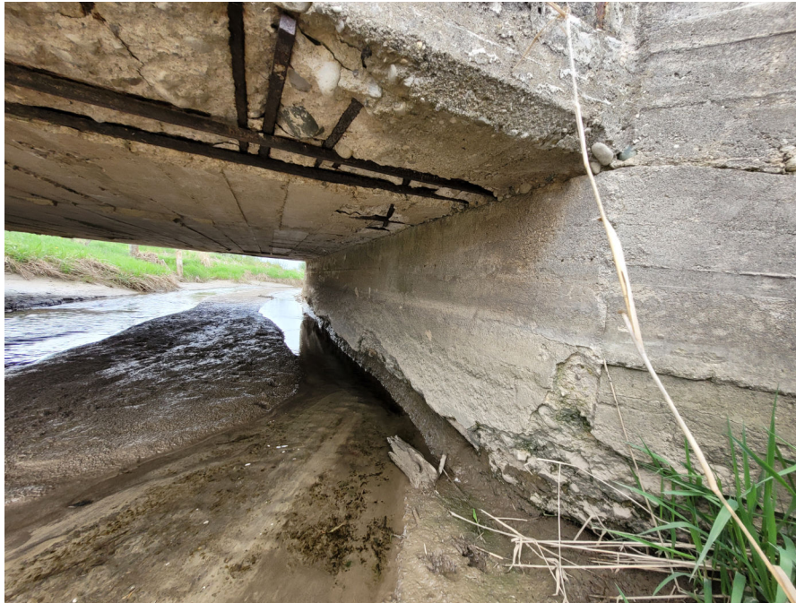
View of abutment wall and soffit, typical.
