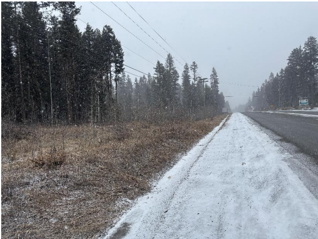
Photograph 6. New access road at junction with Highway 20, looking south towards Williams Lake.
