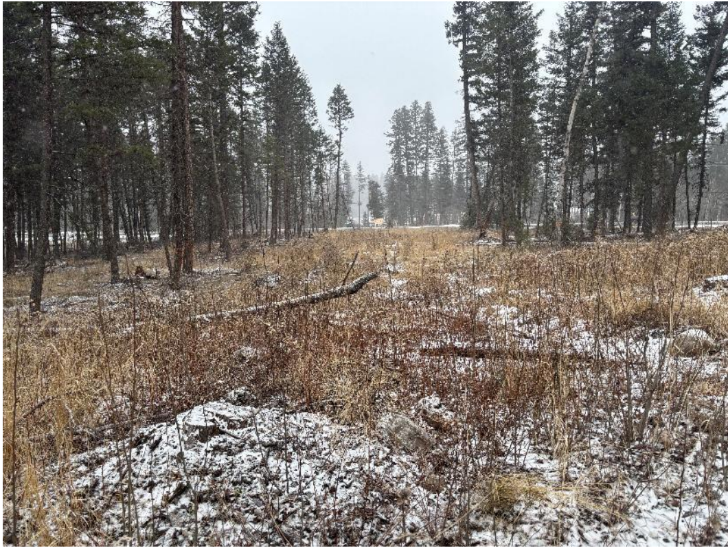
Photograph 5. Final portion of new access road looking at future junction with Highway 20.
