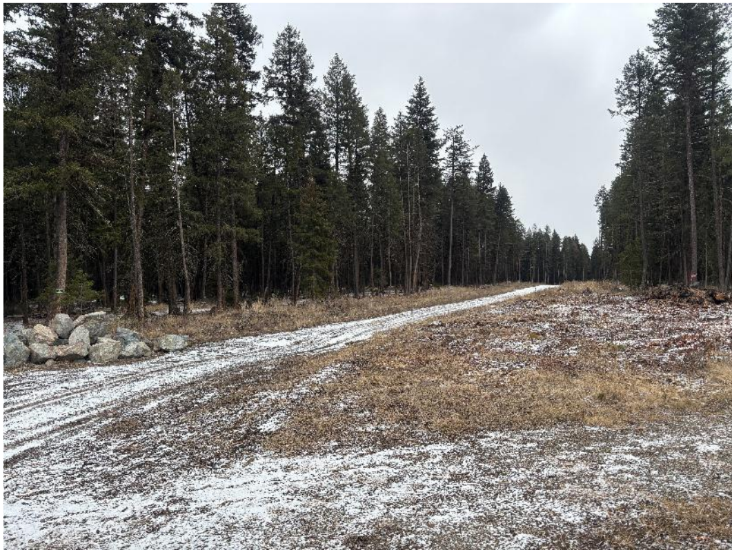
Photograph 3. Existing gravel road and cleared right of way that is part of the new access road to Highway 20.
