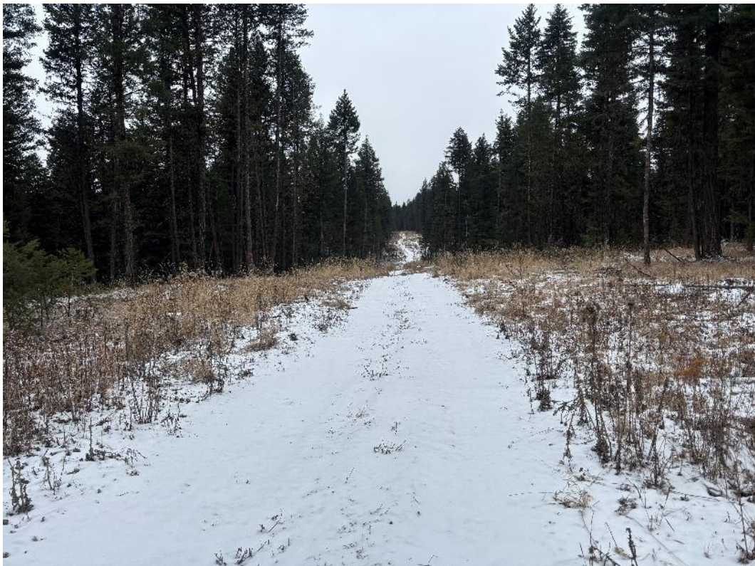
Photograph 4. Middle portion of the new access road to Highway 20 with majority of right of way already cleared.
