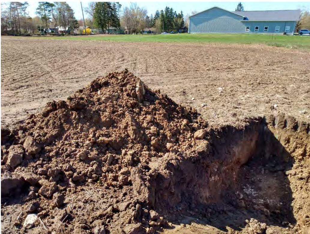
Photo 4: Exposed soil and bedrock in TP8 near the southeast corner of the Site (April 27, 2023).
