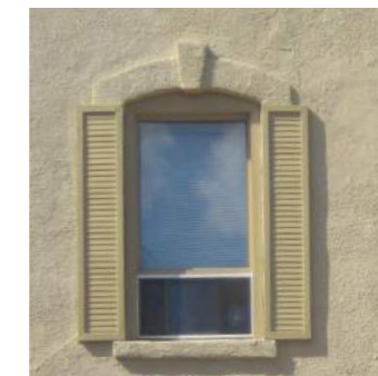
Narrow shutters are not in scale with window width appear inoperable.
