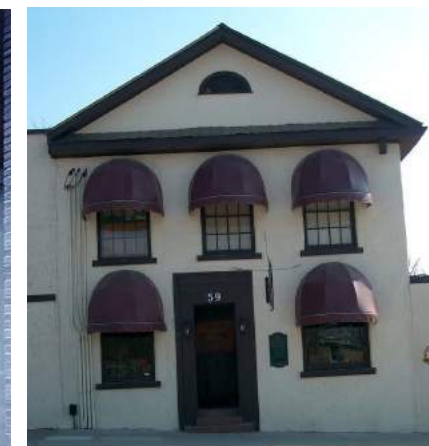
Full stucco facades.
