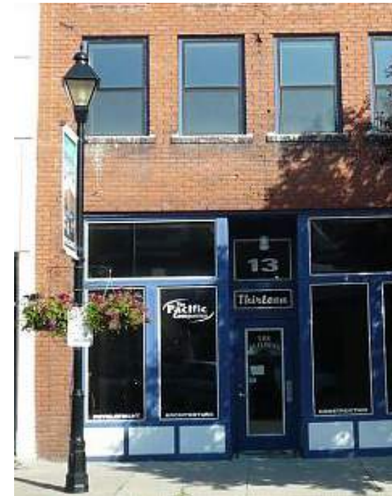
Building entrance flush with sidewalk - barrier-free
