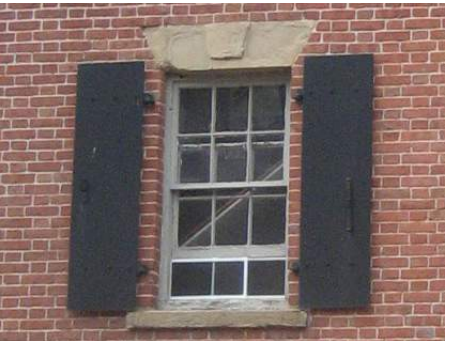
Coloured wooden board shutters with concrete keystone
