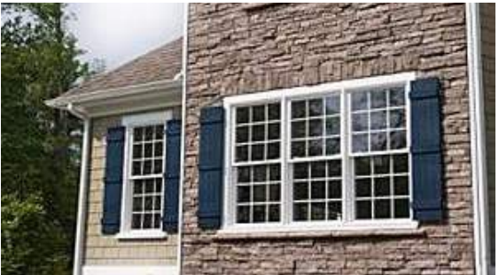
Unrealistic use of shutters.
