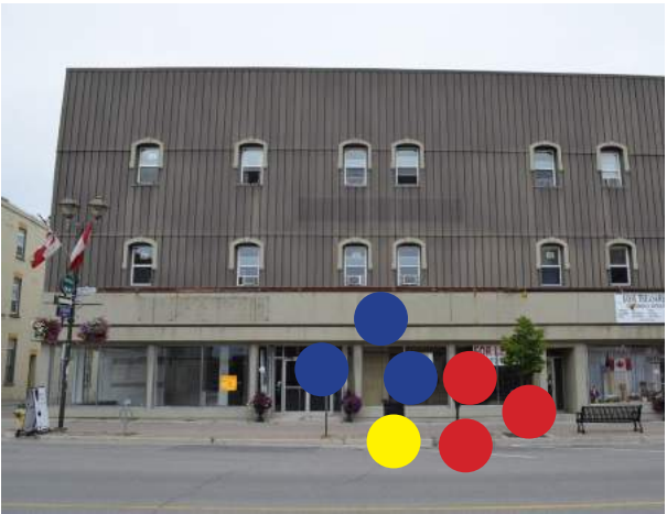
1 Building to Street Dynamic
