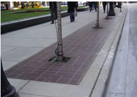
Multiple tree grates optimizes root zone area while maximizing available walkable surface.
