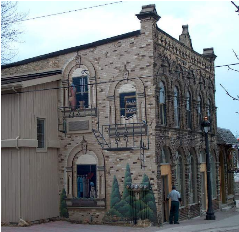
Murals enhancing/ coordinating with existing facades.
