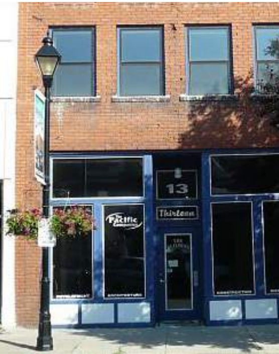
Building entrance flush with sidewalk - barrier-free
