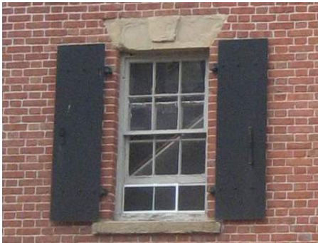
Coloured wooden board shutters with concrete keystone
