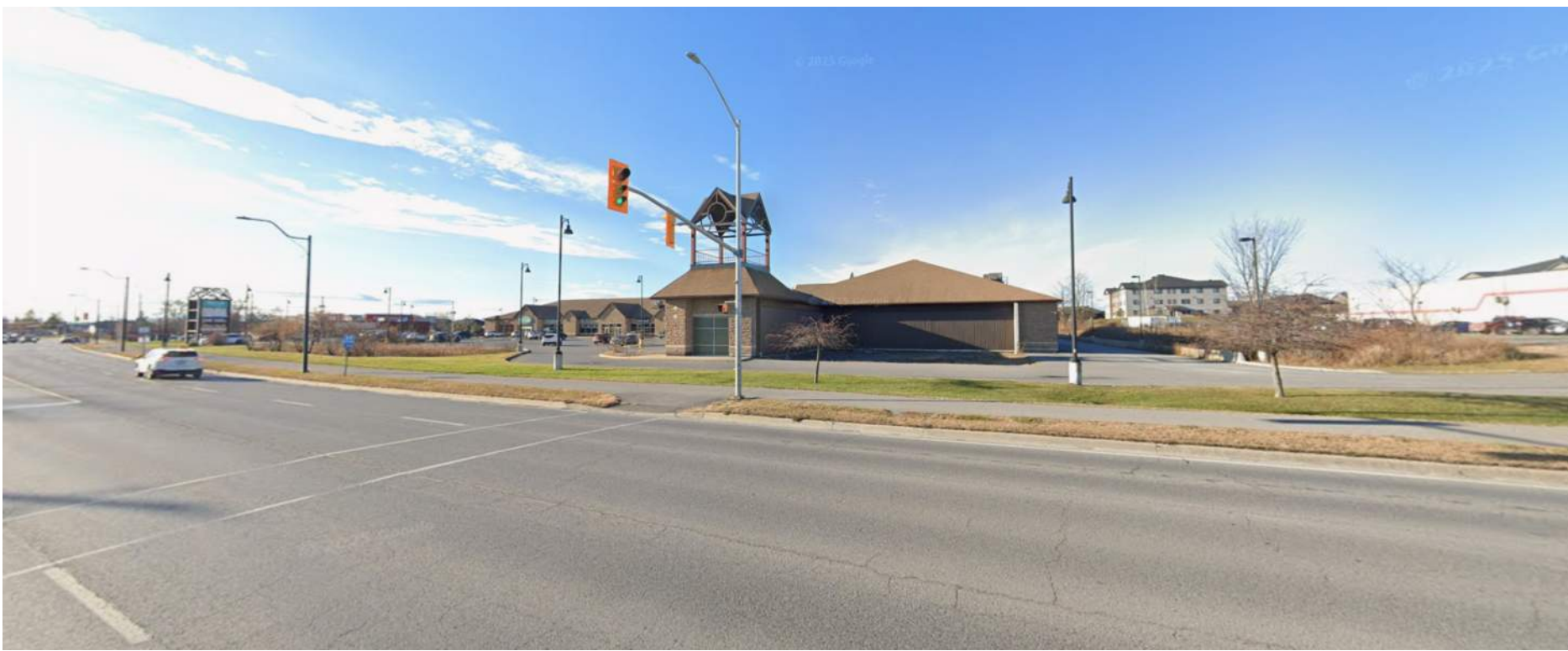
2. VIEW FROM OTTAWA STREET - LOOKING NORTH WEST
