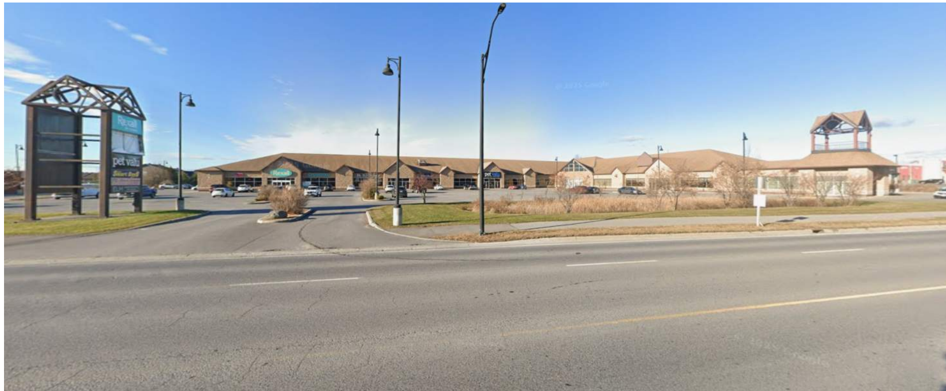
1. VIEW FROM OTTAWA STREET - LOOKING NORTH
