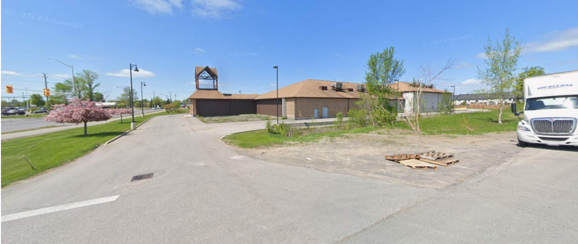
4. VIEW FROM ADJACENT SITE - LOOKING SOUTH WEST
