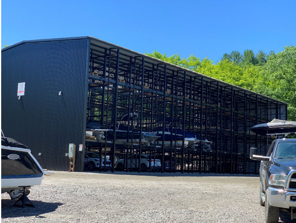
Figure 3: Boat Storage Building
