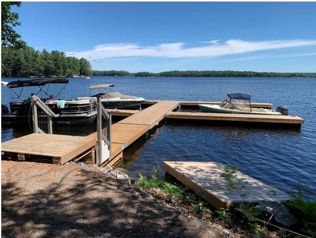
Figure 4: Existing Dock 'E'
