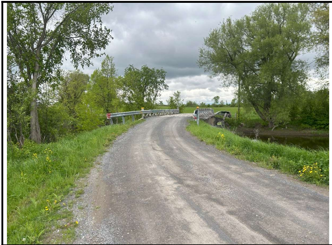
Photo 2 Structure from South approach
