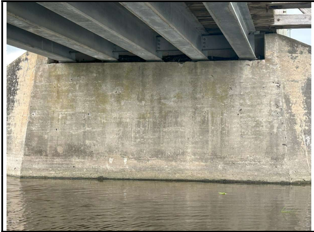
Photo 13 Typical view of north abutment wall
