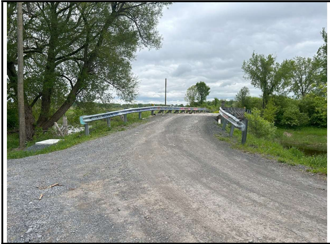
Photo 1 Structure from North approach
