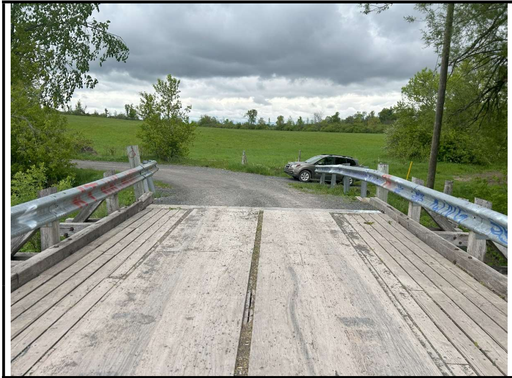
Photo 3 North approach from center of structure
