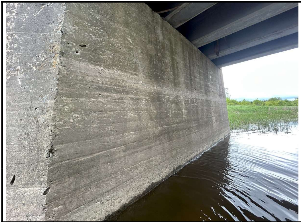
Photo 14 Typical view of south abutment wall
