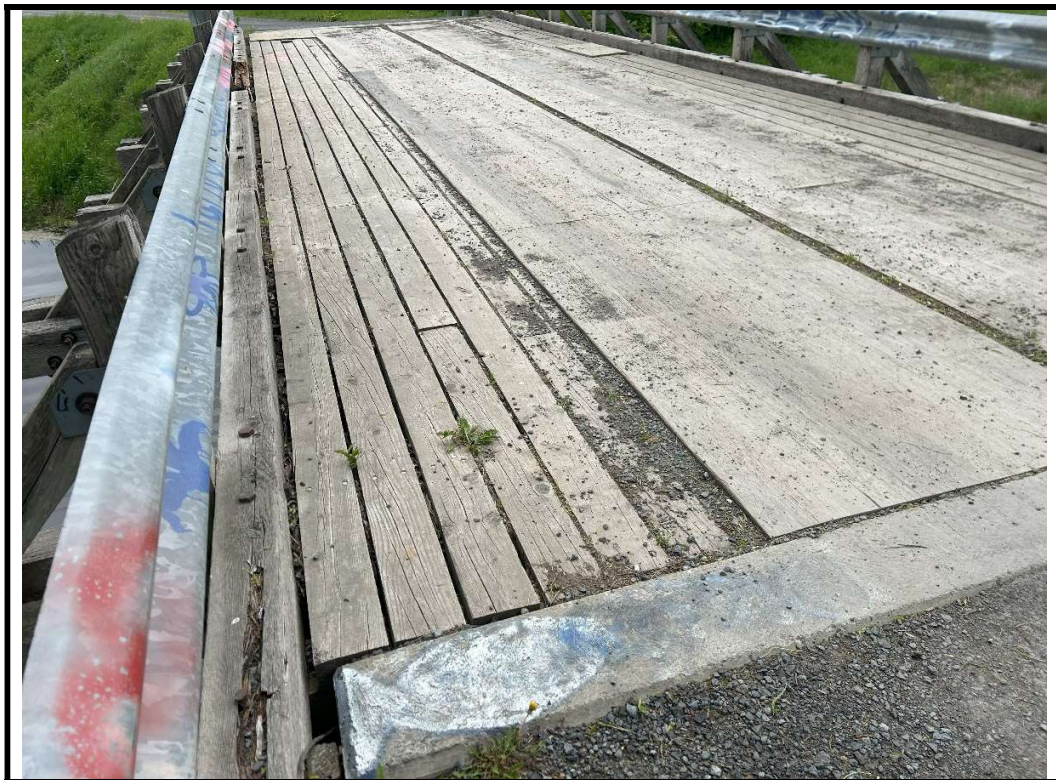
Photo 10 Typical view of deck top
