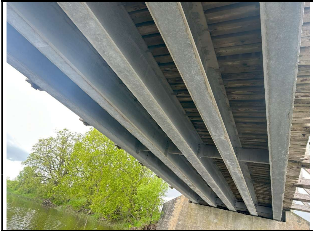
Photo 15 Typical view of deck underside
