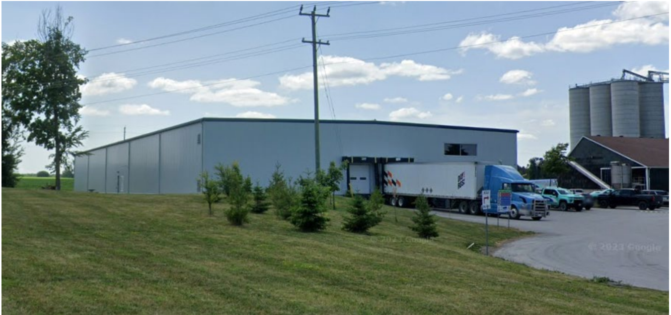
Figure 5. Existing warehouse building on the subject property
