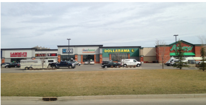
Existing commercial uses adjacent to Highway 27.
