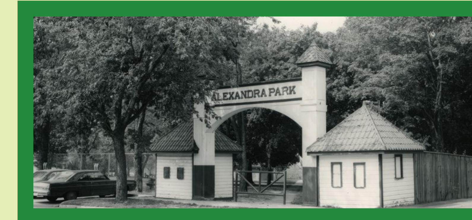
Alexandra Park gates on what was Alexandra Street, now Hospital Court. Source: Oshawa Museum, archival collection.
