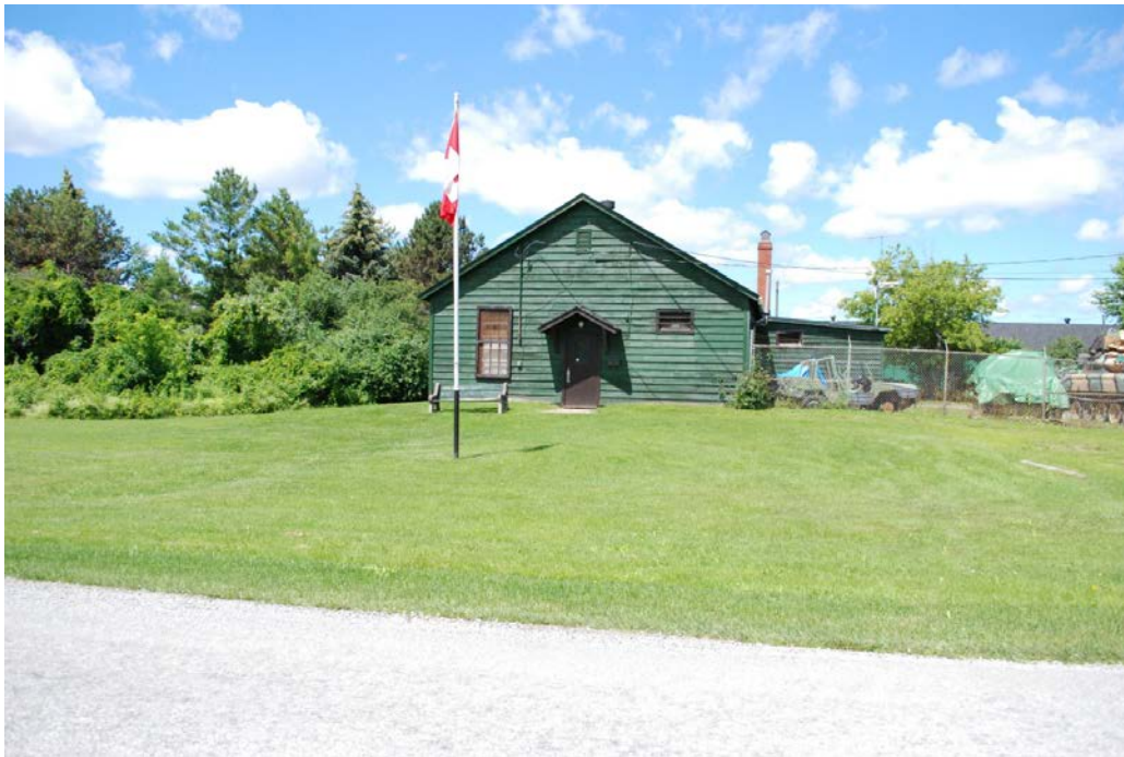
6. East Facade, Former Stores Building
