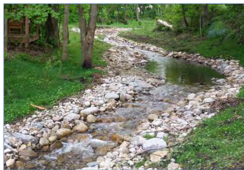
An example of natural channel design with riffle-pool morphology
