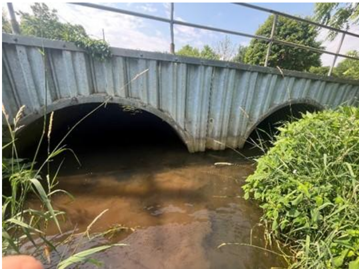
Figure 5-8: York Street Culvert Looking Downstream
