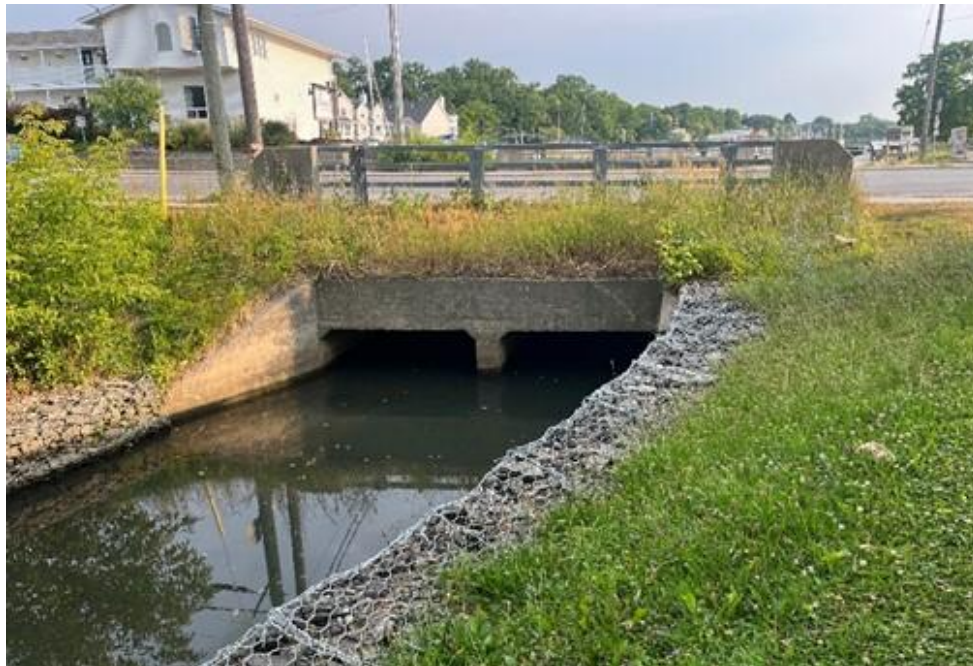
Figure 5-10: Bridge Street Culvert Looking Downstream
