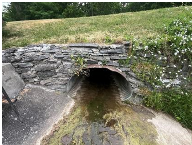
Figure 5-2: Church Street Culvert Looking Upstream
