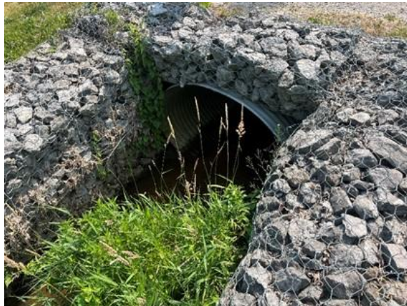
Figure 5-6: Lalor Street Culvert Looking Upstream
