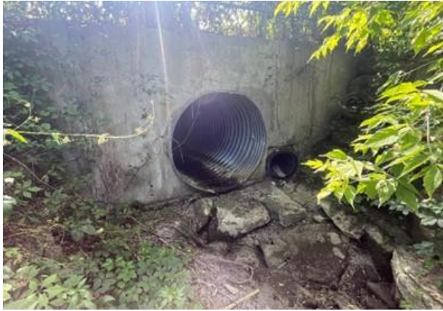
Figure 5-4: Pitt Street Culvert Looking Upstream
