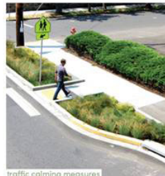
traffic calming measures
