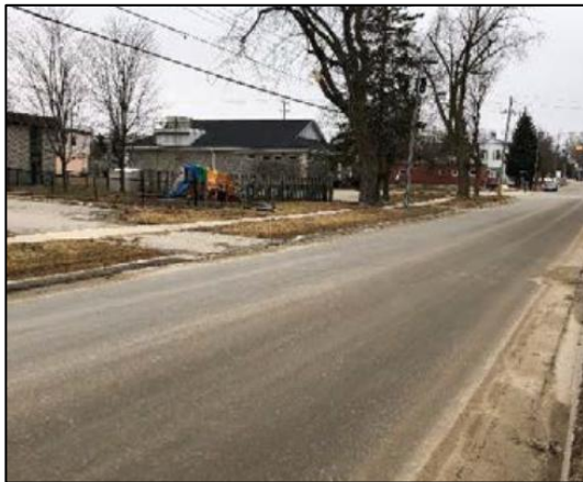
Figure 11-11: Good Condition (PCR 70 - 85)
