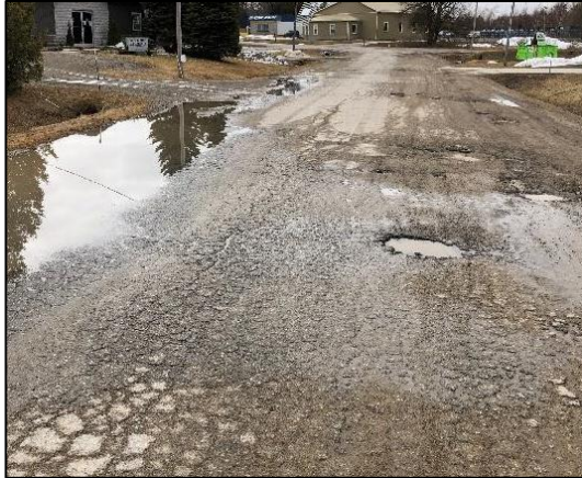
Figure 11-9: Poor Condition (PCR < 60)
