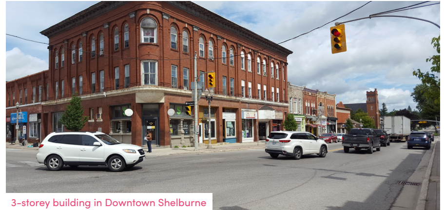
3-storey building in Downtown Shelburne
