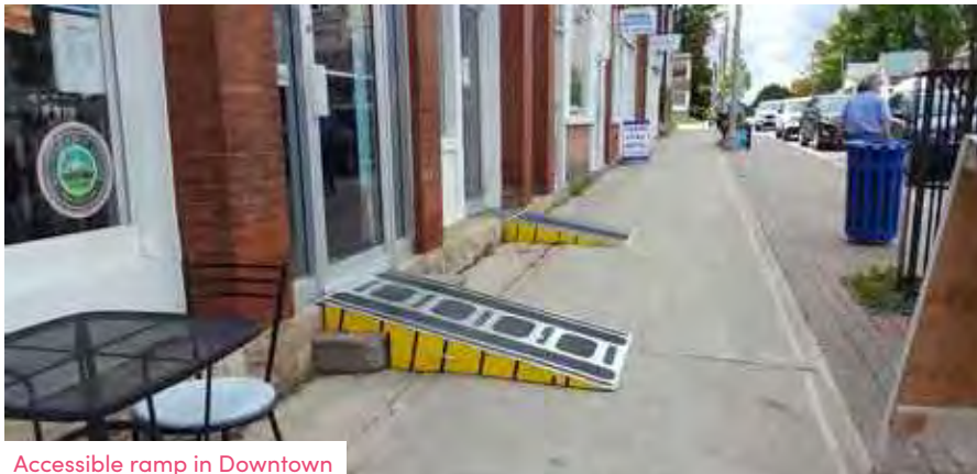
Accessible ramp in Downtown
