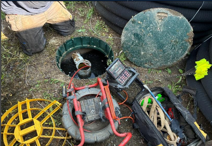
7. Camera inspection of discharge line – leading from septic tank to leaching field
