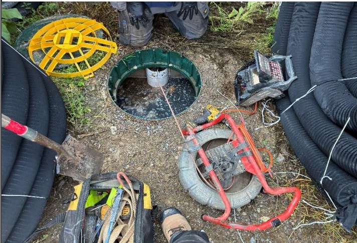
3. Camera inspection of sewer line
