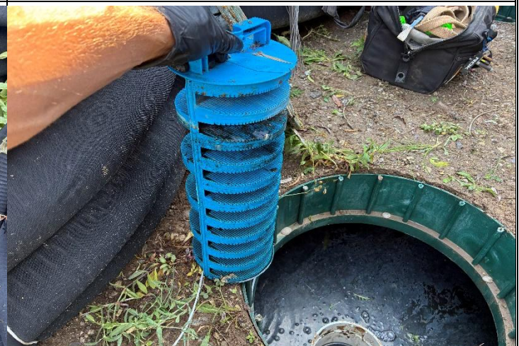
6. Effluent filter installed in outlet compartment of tank – removed and cleaned during inspection
