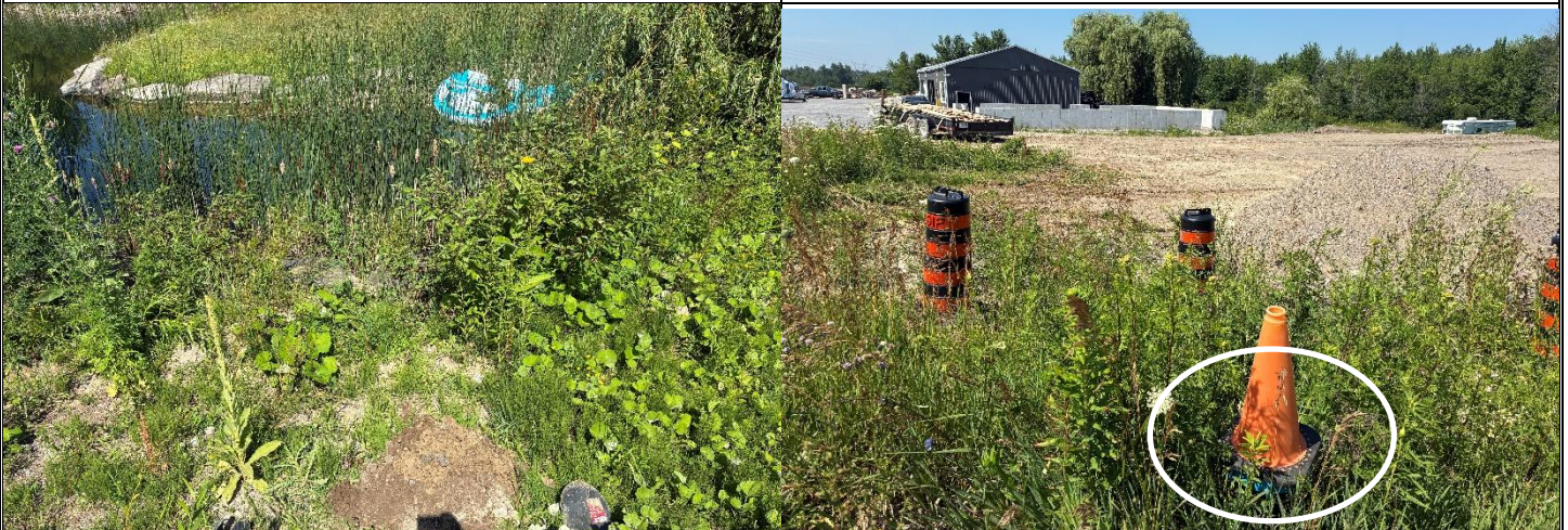
21. Location of test hole 2 located at the end of the sand filter bed mantle
