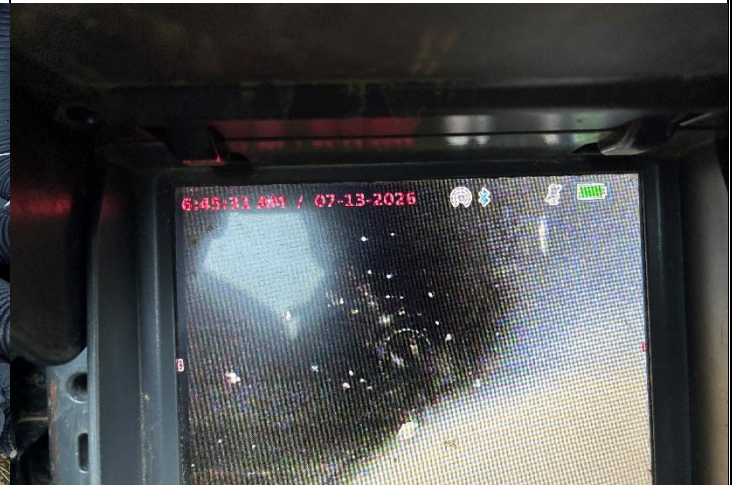
4. Interior of sewer line
