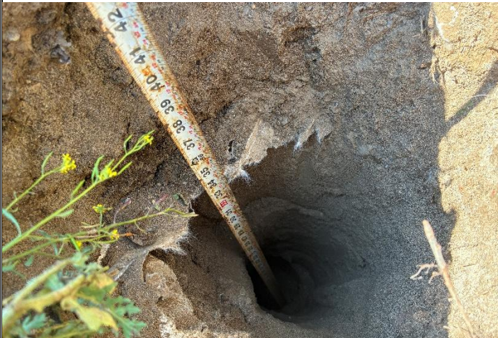
15. Interior of test hole 1. No water observed and geotextile covering washed stone visible
