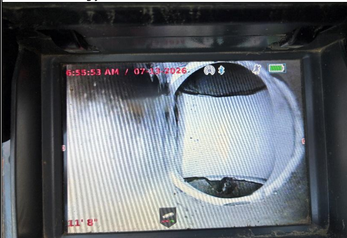
9. Interior of discharge line – header manifold visible
