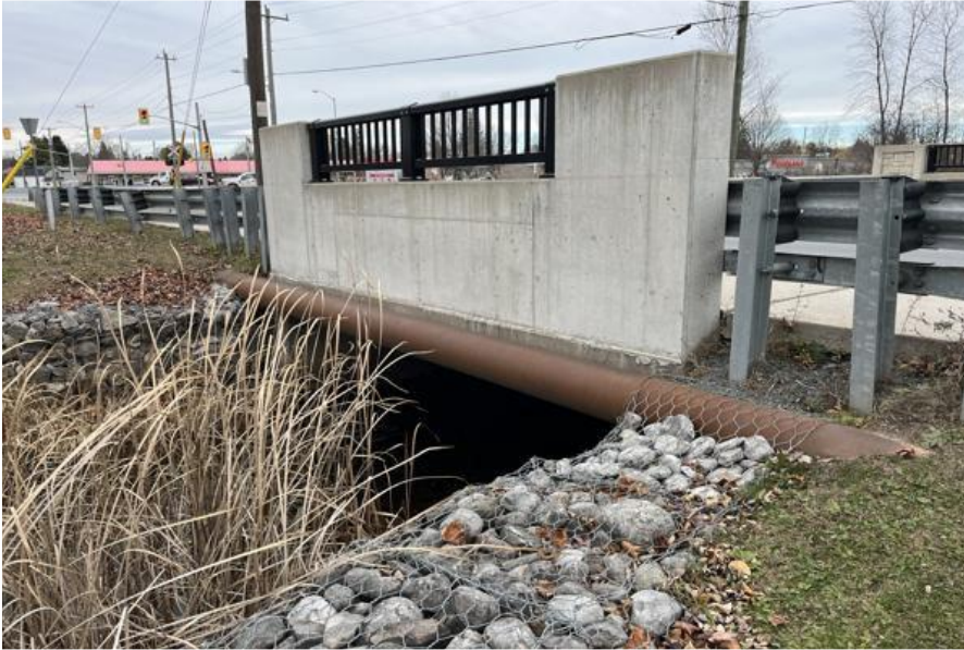
Figure 85 Bridge in Good Condition Example
