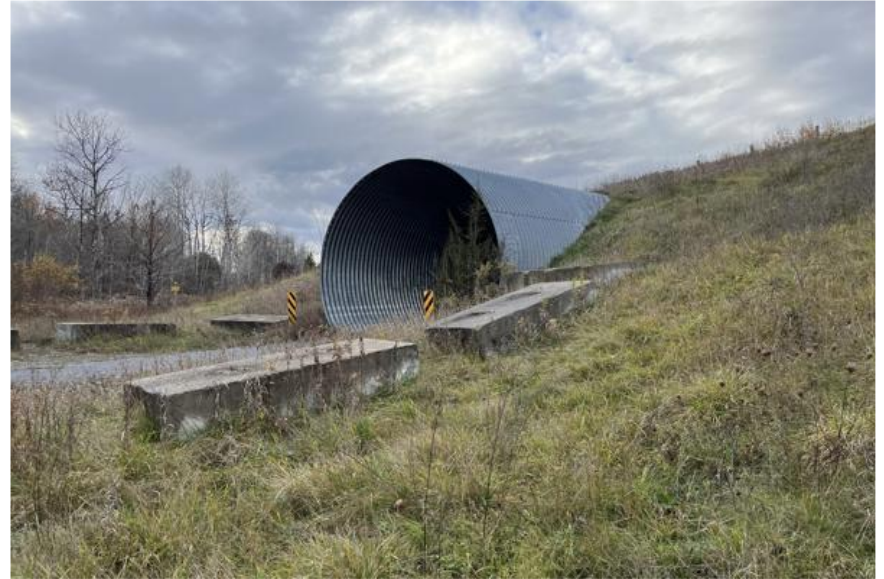
Figure 86 Culvert in Good Condition Example
