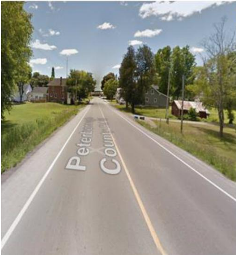
Figure 82 Road Surface in Good Condition Example
