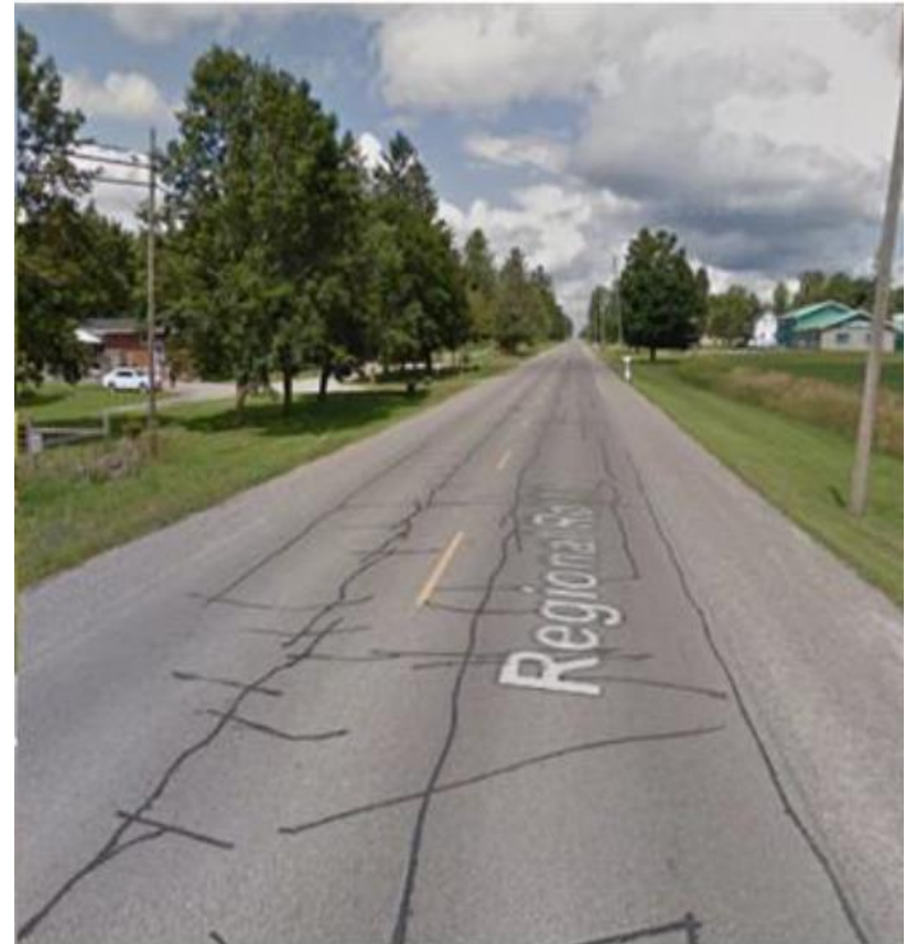
Figure 83 Road Surface in Fair Condition Example
