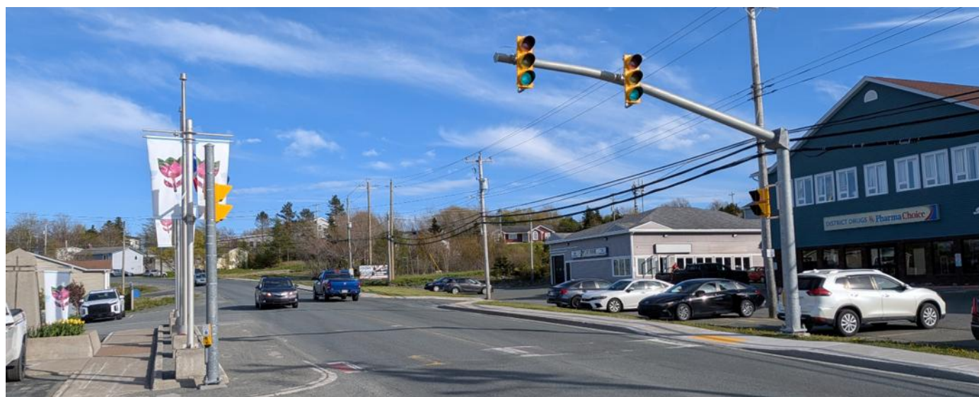
Figure 26: Traffic Signal (TS) Crosswalk
