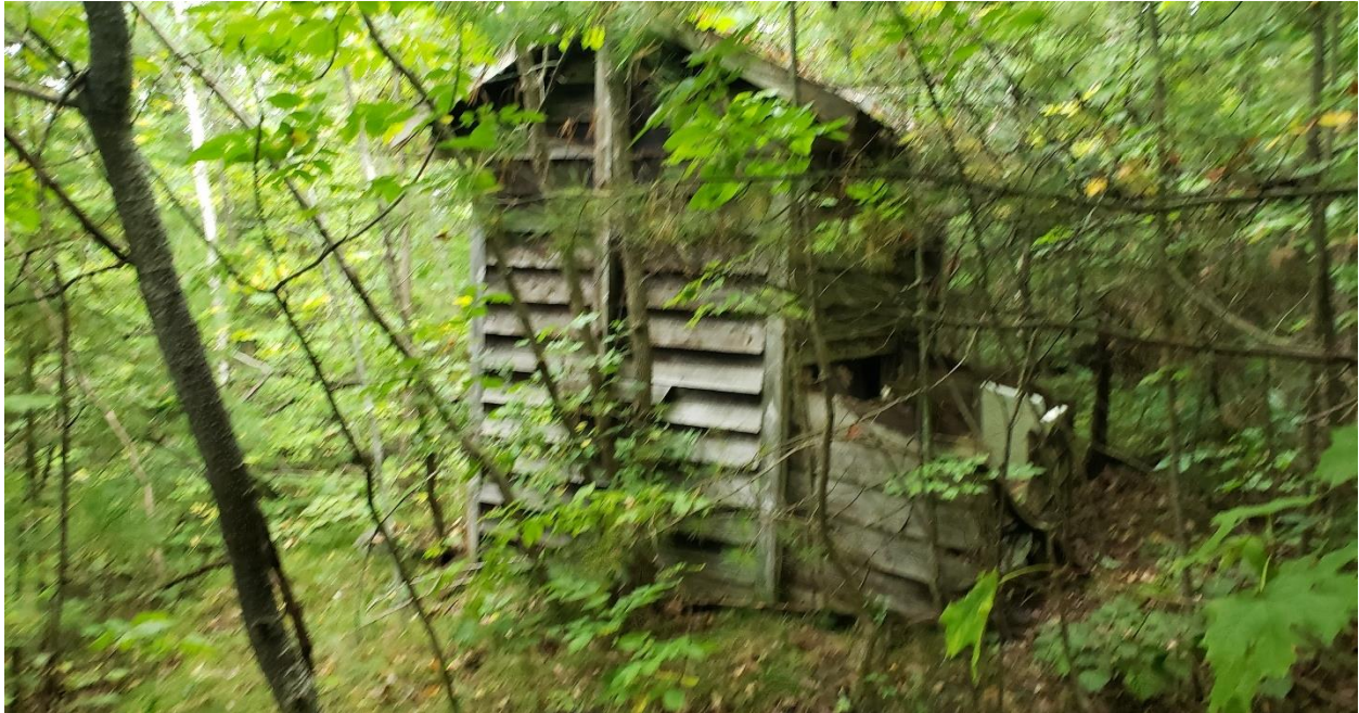
Image 9.7: Oriented E- View of The Standing Pump House.
