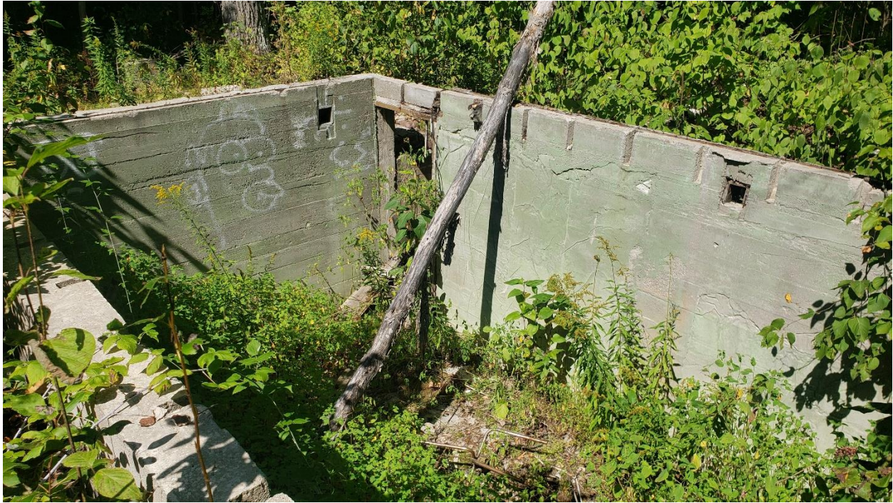
Image 9.5: Oriented S- View of The Dug-out Foundation of the Removed Cottage, Demolition Occurred Prior to the Assessment.
