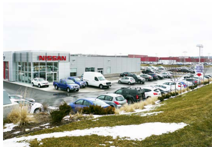
Figure 6-2. Northfield Drive contains a number of car dealerships with parking areas that front onto the street.
