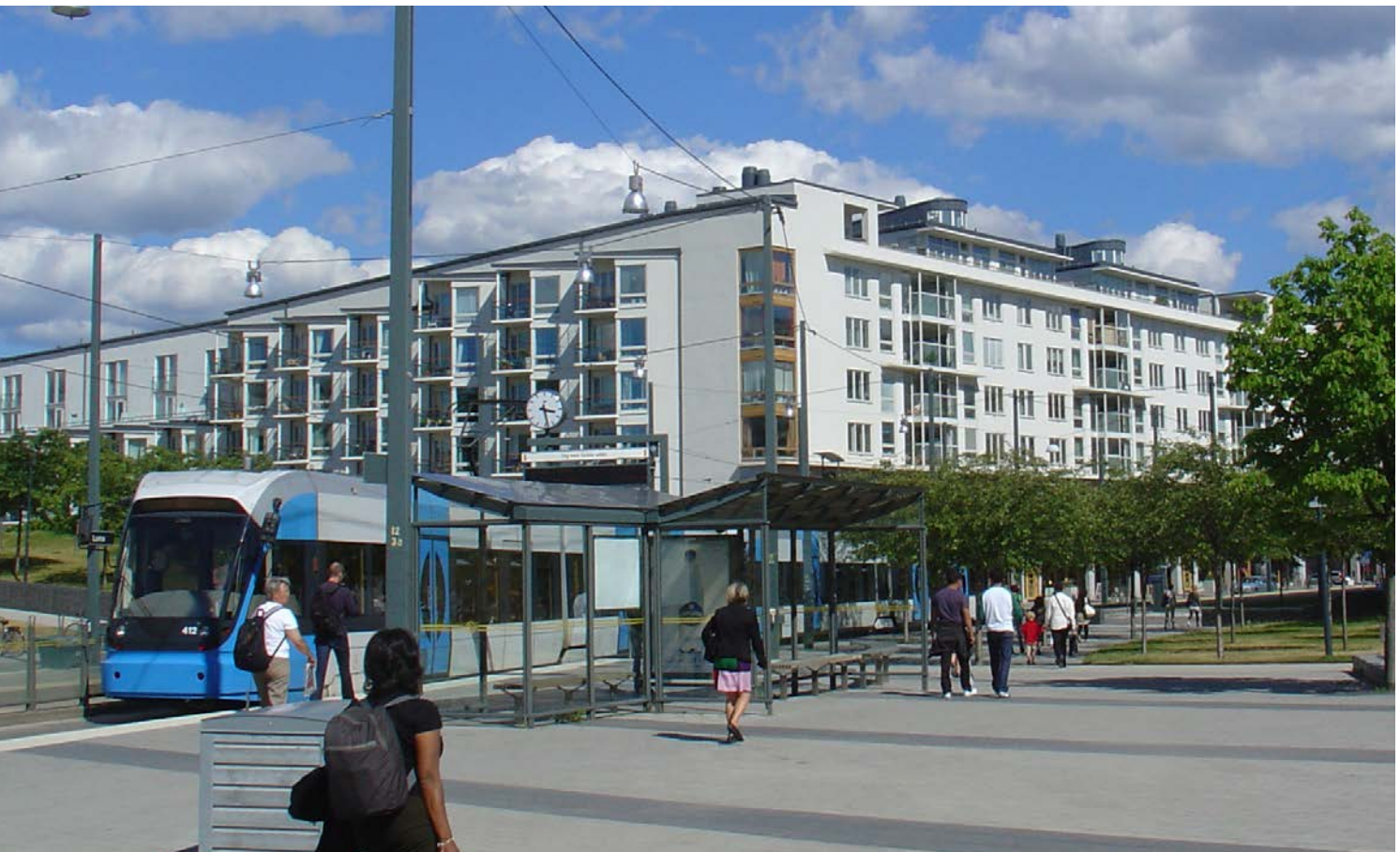
Figure 2-6. By locating more active uses next to the stations and integrating the stations with the community's open space network, Stockholm's Hammarby Sjostad neighbourhood promotes higher levels of activity around its LRT stations.
