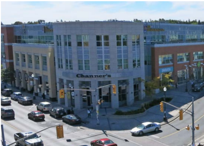
Figure 5-11. The integration of amenities in the ground floor of this office building in Uptown Waterloo helps to animate the street and support local employees
