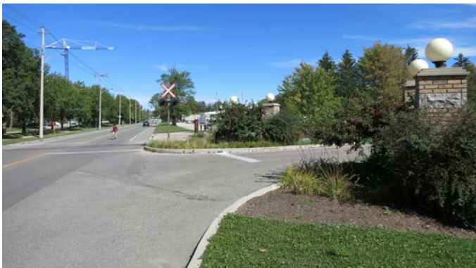
Figure 3-3. Seagram Drive is an important connection linking the station with Wilfrid Laurier University and the University of Waterloo
