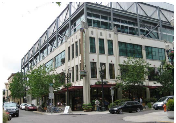
Figure 5-13. Buildings with active frontages can provide amenities and support active street level uses (Portland, Oregon)
