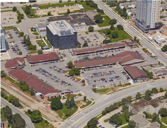
Figure 4-16. Bird's eye view of the University Shops Plaza, consisting of single-storey retail pads and surface parking areas
