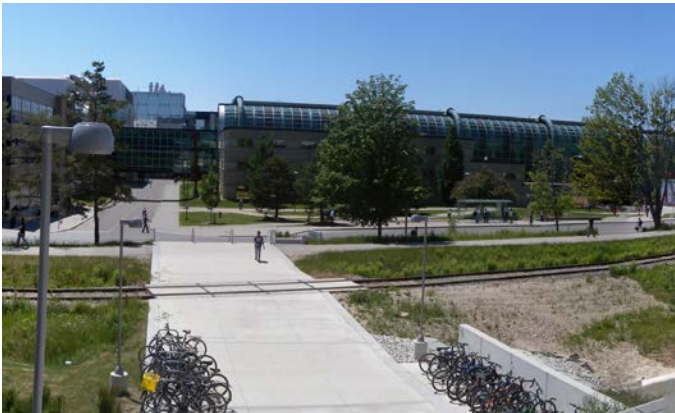
Figure 4-2. Many of the University's building are oriented away from the station just east of the Ring Road
